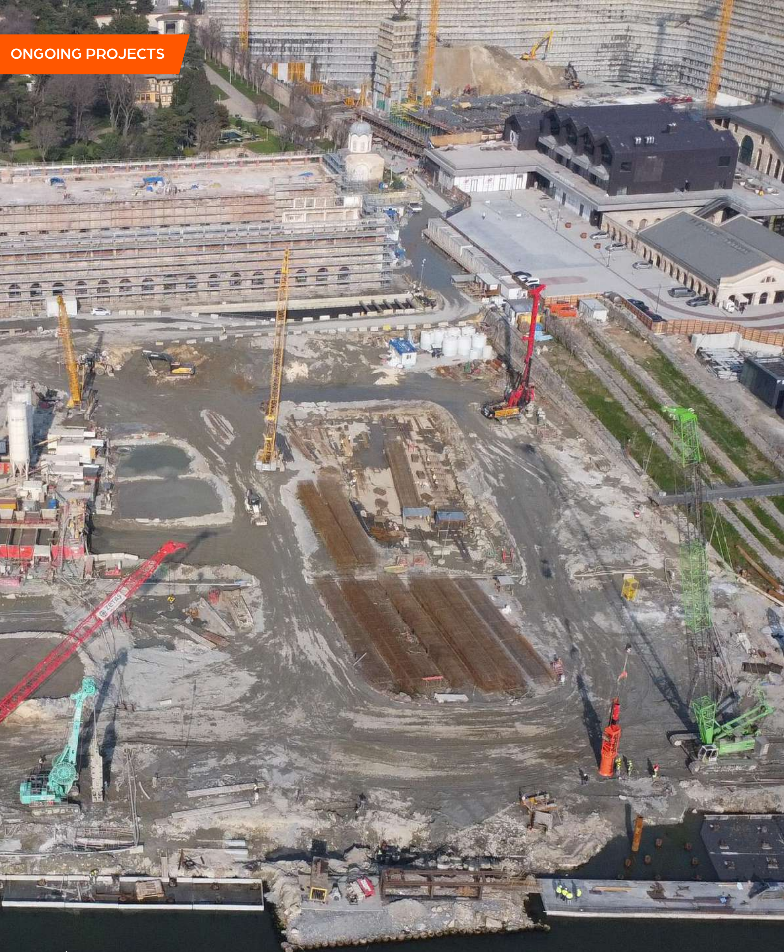
Project Name: Tersane Istanbul Zone-6 Piled Wharf Construction
